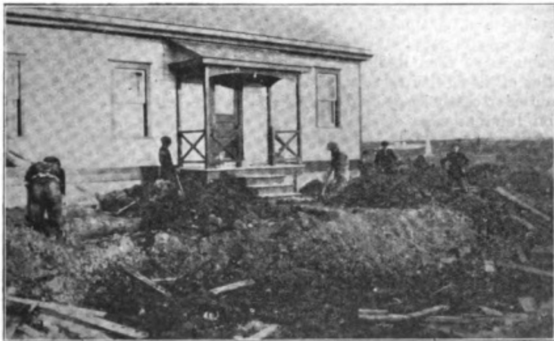
Erecting the Kingston Station Building.
