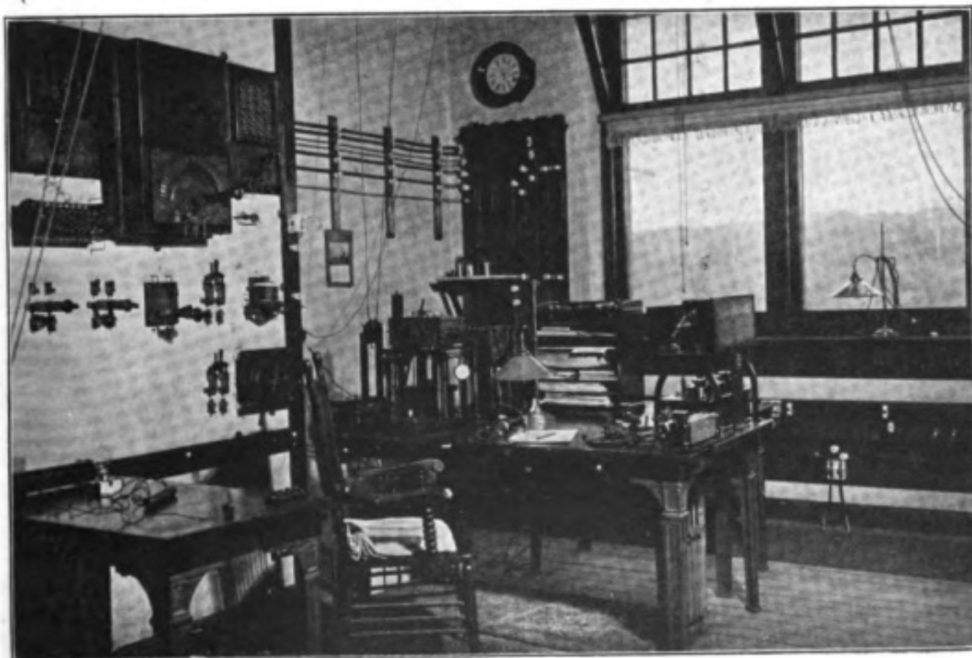
The Interior of the Operating Room.
