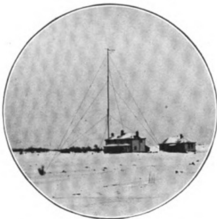
The Kingston Station, Buildings and Mast.
